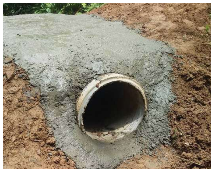
Installed culvert to channel surface run-off during heavy downpour
