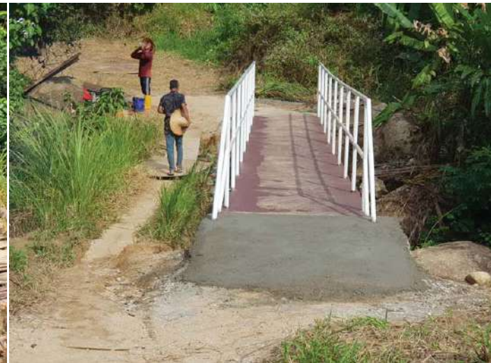
The completed bridge to connect Kampung Sagong
