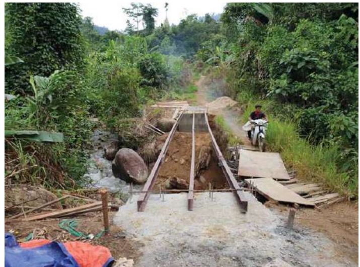
The primary steel frame of the bridge was laid down
